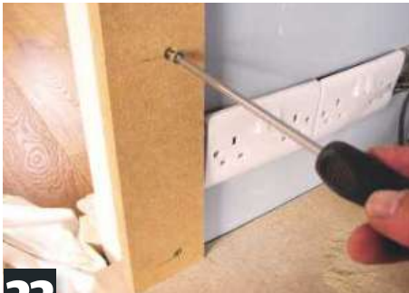
22 Door hinges are fixed to 19mm MDF uprights. Fix these securely to walls with 5mm screws
